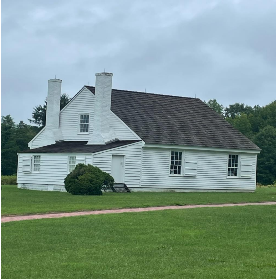
Photograph 1 - Jackson Shrine Death Site house structure.
