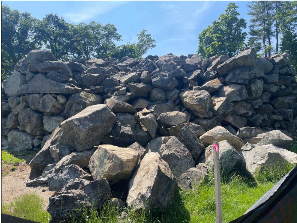
Example of Collapsed Section - Rock Formation
