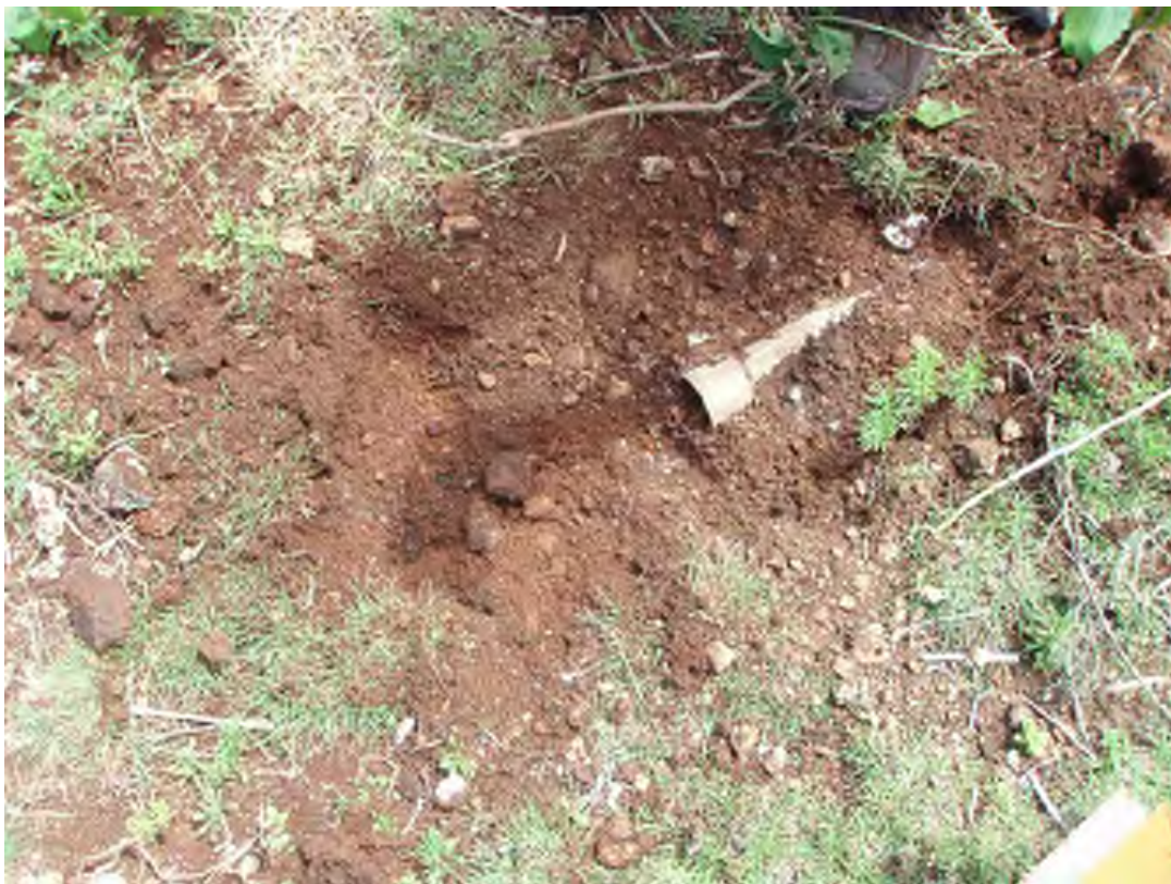
Figure A.10. Subsurface pipe located at Site 78, Andersen AFB, Guam
