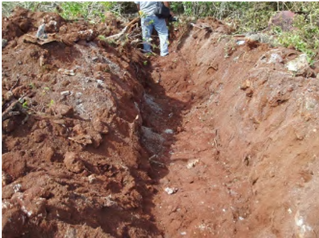
Figure A.12. Trench TT-03 at Site 78, Andersen AFB, Guam
