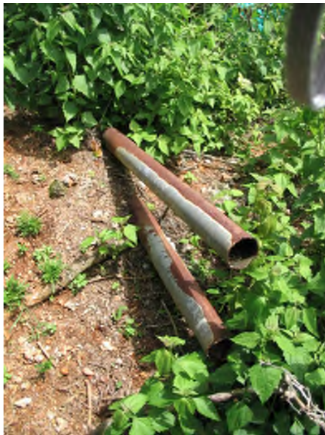
Figure A.8. Pipes located at Site 78, Andersen AFB, Guam
