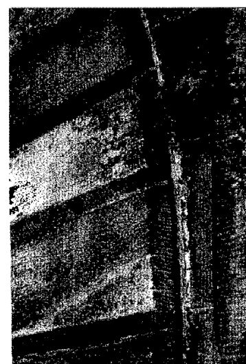
8 A7 DETAIL OF ARCH VOUSSOIRS & SPANDREL STONES, WEST PORTAL
