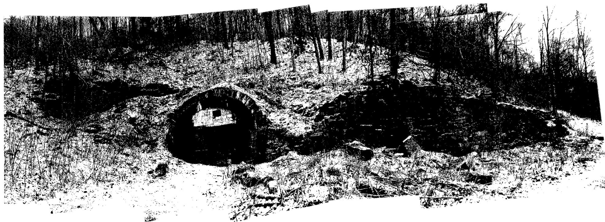
2 OVERALL VIEW OF EAST PORTAL AREA N.T.S.
