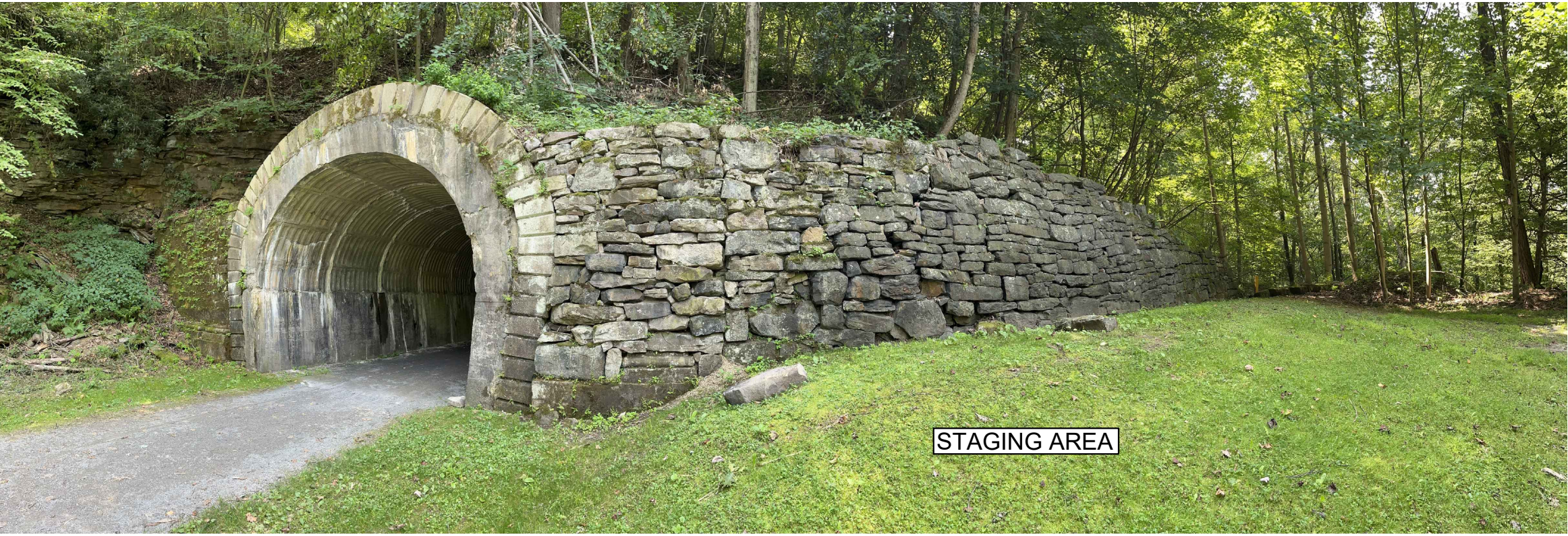
NORTH TUNNEL ENTRANCE
