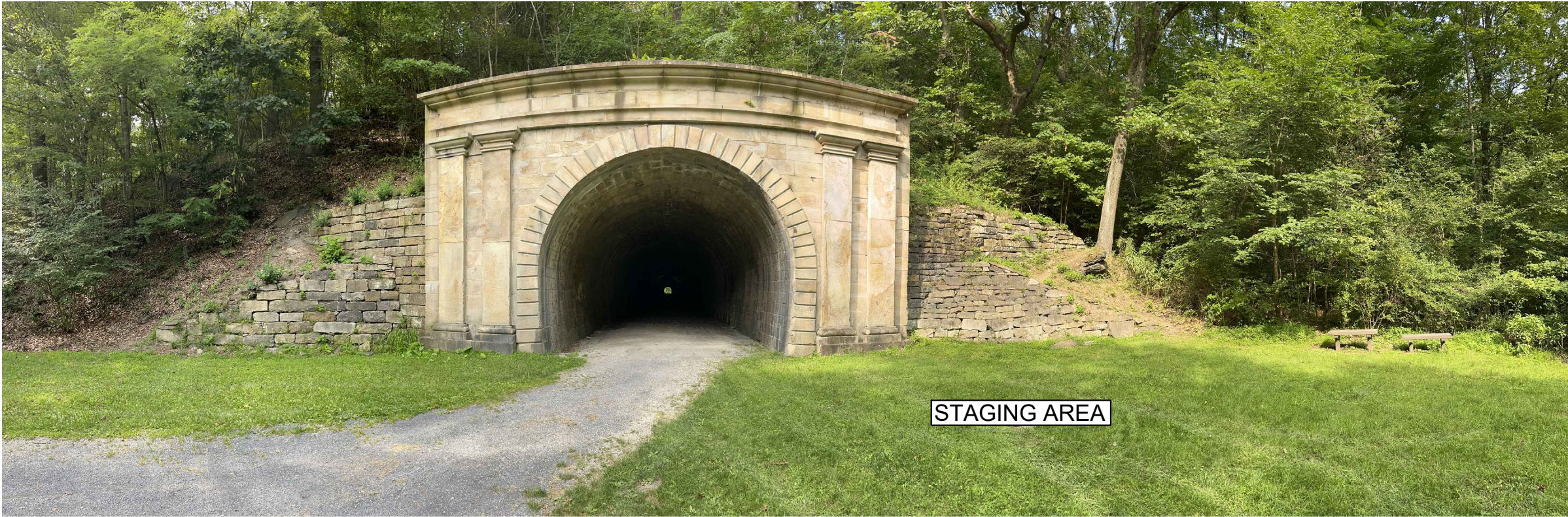
SOUTH TUNNEL ENTRANCE
