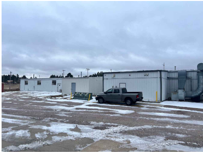
PH2 A0.1 EXISTING CONDITIONS NO SCALE
