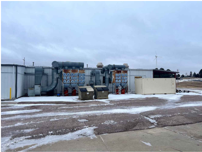
PH1 A0.1 EXISTING CONDITIONS NO SCALE
