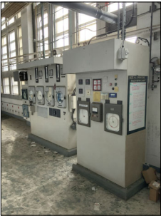
37 G37 - BOILER AREA SCALE: NO SCALE REF DWG: G1004
