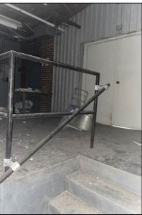
45 G45 - BOILER RM 108 SCALE: NO SCALE REF DWG: G1004
