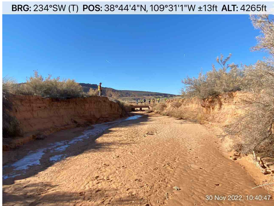
Upstream of Winter Camp Wash
