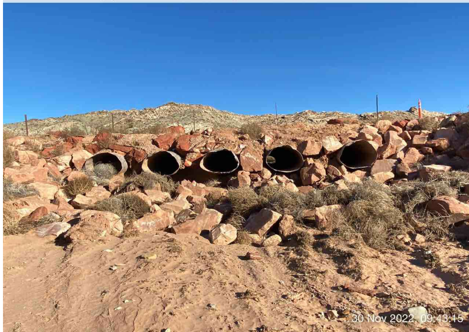
Outlet of Salt Valley Wash
