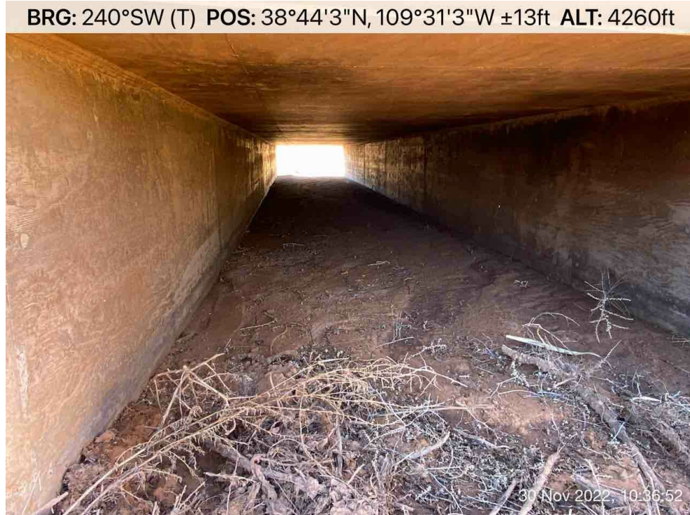
Condition of Existing Culvert
