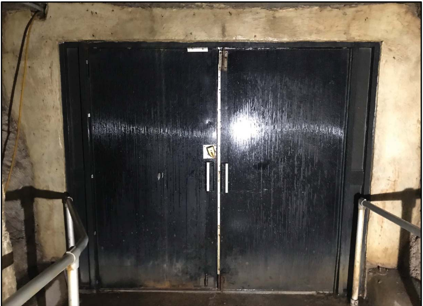
Figure 25: Dripstone Cave Exit - Security Doors (Existing Conditions)
