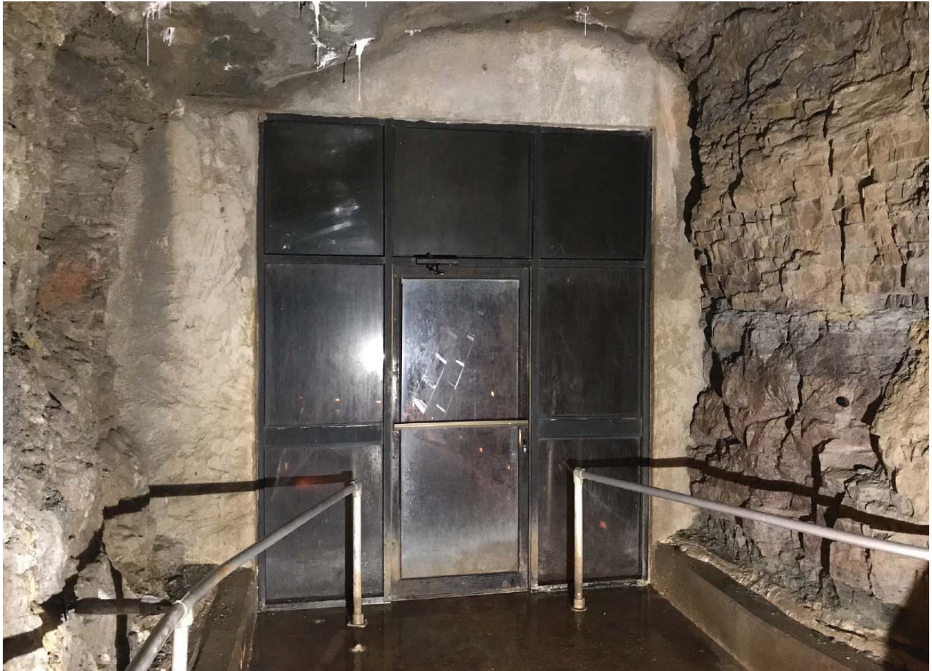
Figure 28: Discovery Cave Exit – Inner Airlock Door (Existing Conditions)
