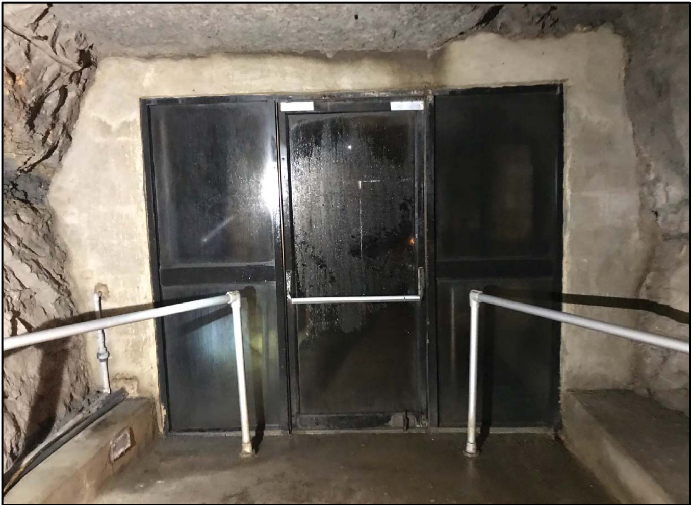
Figure 24: Dripstone Cave Exit – Outer Airlock Door (Existing Conditions)
