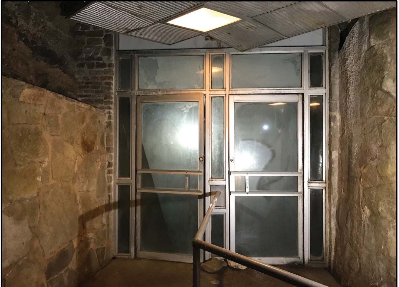
Figure 20: Dripstone Cave Entrance – Outer Airlock Doors (Existing Conditions). Existing stacked stone masonry bulkhead visible on left side of doors.
