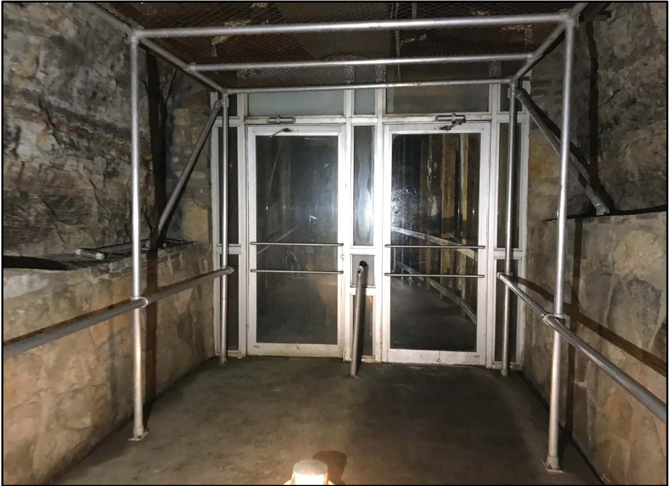
Figure 21: Dripstone Cave Entrance – Inner Airlock Doors (Existing Conditions)
