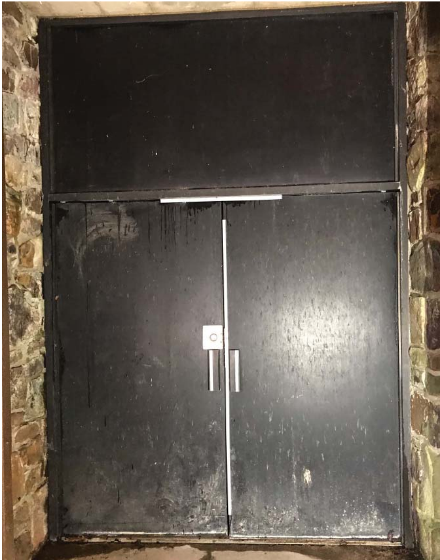
Figure 26: Discovery Cave Exit - Security Doors (Existing Conditions)
