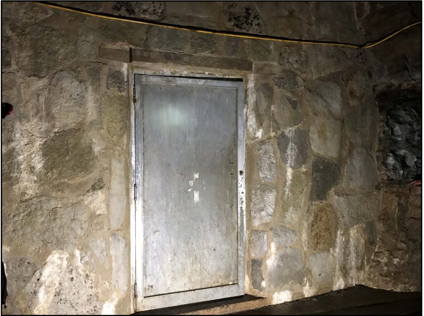
Figure 22: Dripstone Cave Bypass Tunnel Door (Existing Conditions)
