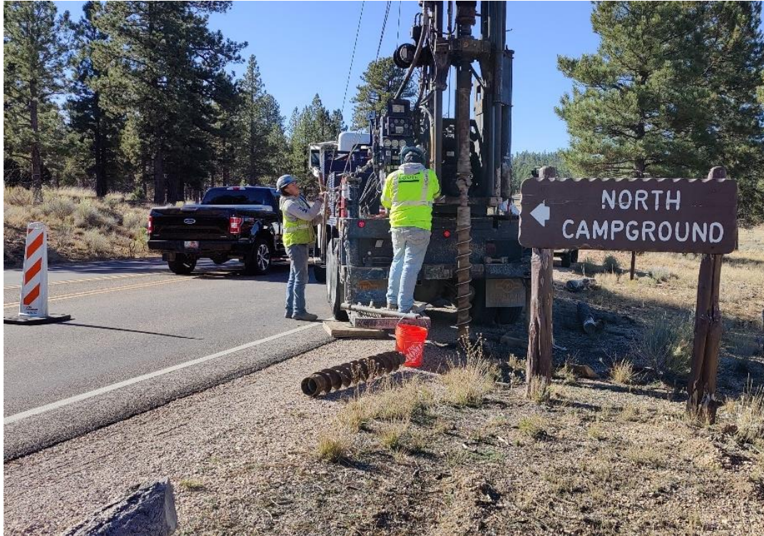
YA-B5 – Pavement in good condition – shoulder boring
