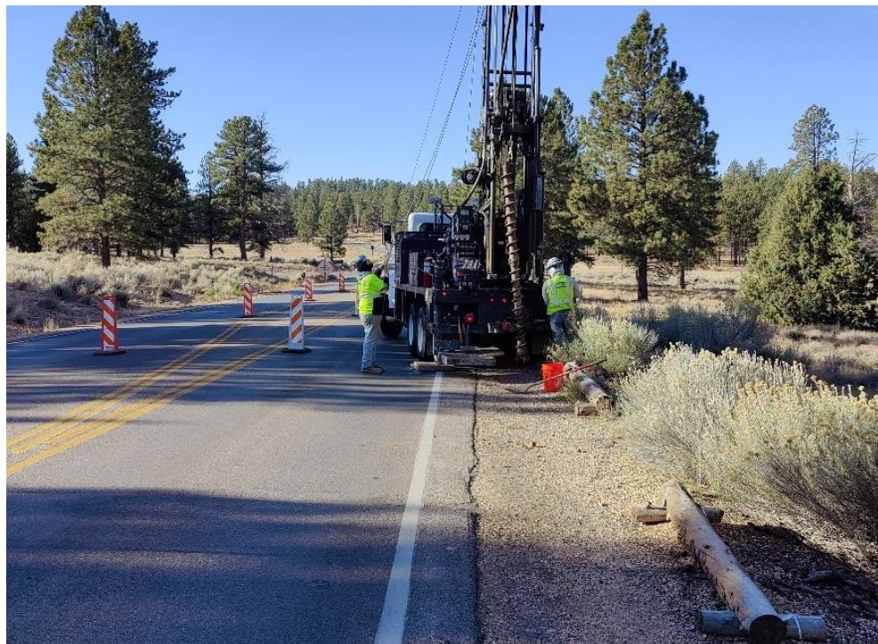
YA-B4 – Pavement in good condition - shoulder boring
