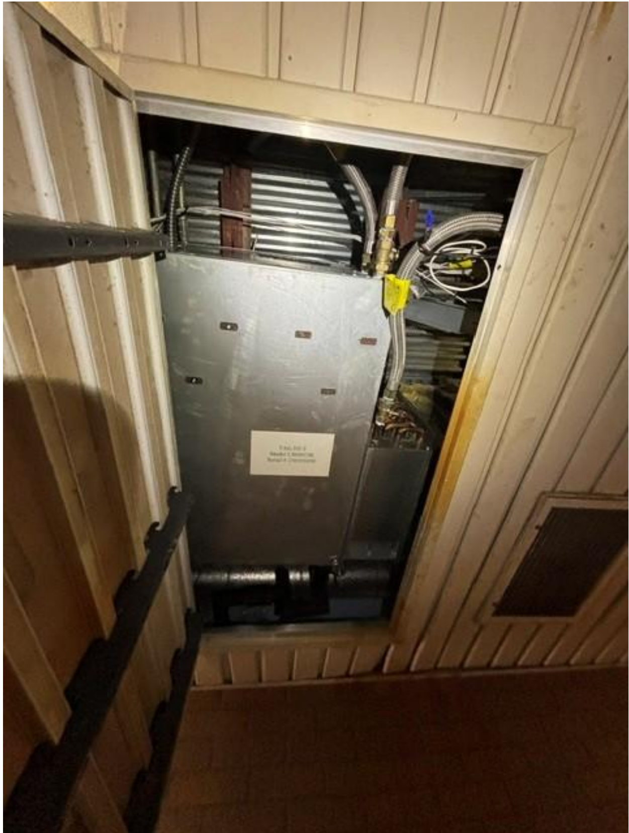
DOAS: Corridor Access – Open Hatch
