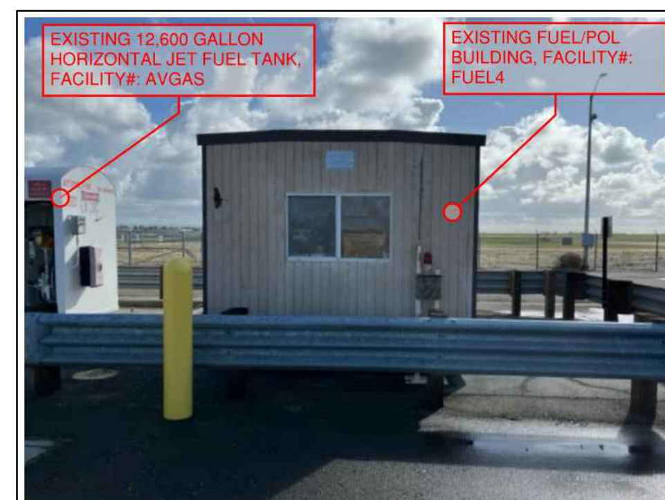
L10 EXISTING FUEL/POL BUILDING (LOOKING EAST) SCALE: NO TO SCALE
