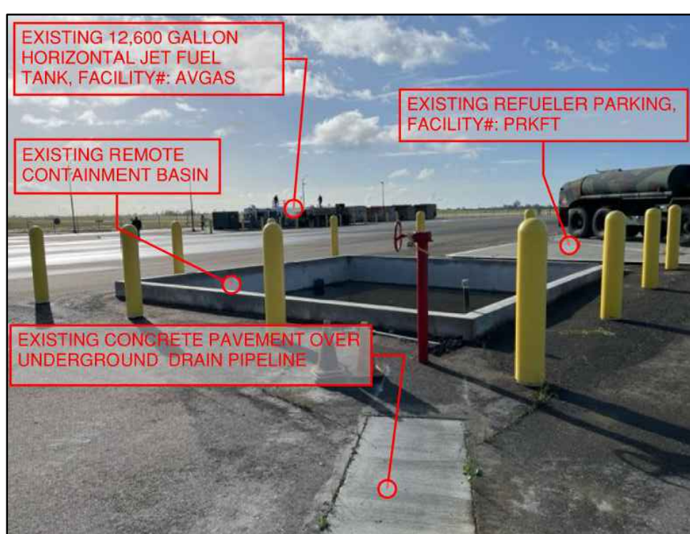
A1 EXISTING CONCRETE PAVEMENT OVER UNDERGROUND DRAIN PIPELINE BETWEEN RCB AND DRAIN INLET (LOOKING SOUTHEAST) SCALE: NOT TO SCALE
