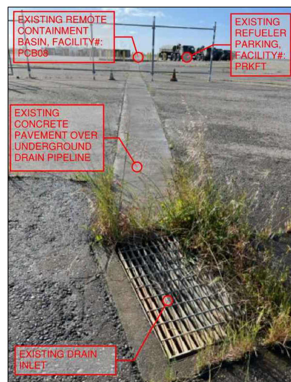
A10 EXISTING CONCRETE PAVEMENT OVER UNDERGROUND DRAIN PIPELINE BETWEEN RCB AND DRAIN INLET (LOOKING SOUTHEAST) SCALE: NOT TO SCALE
