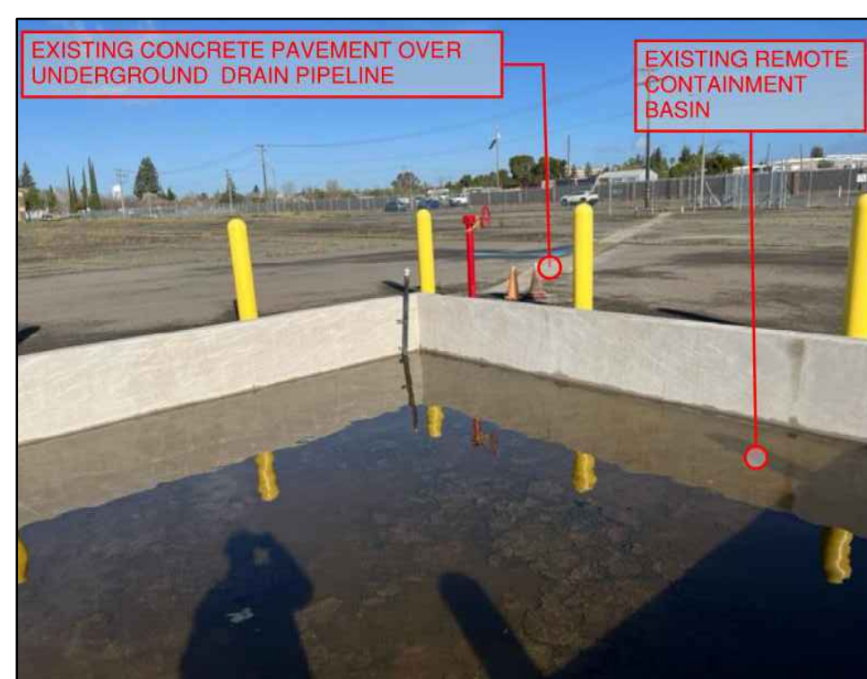
G1 EXISTING CONCRETE PAVEMENT OVER UNDERGROUND DRAIN PIPELINE BETWEEN RCB AND DRAIN INLET (LOOKING NORTHWEST) SCALE: NOT TO SCALE
