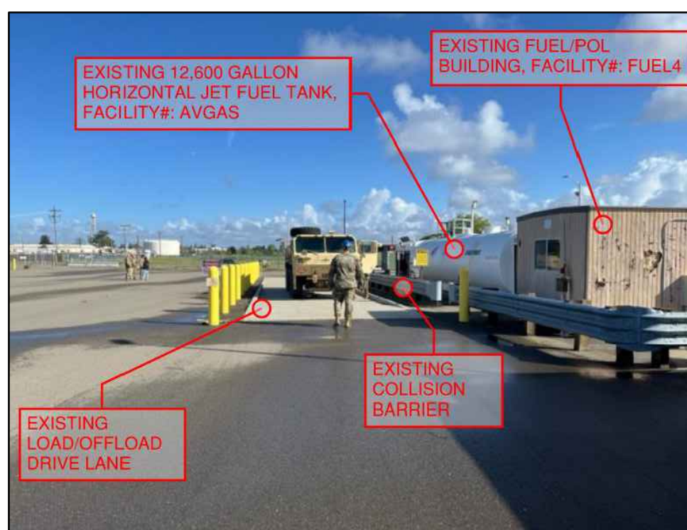
L1 EXISTING FUEL/POL BUILDING (LOOKING NORTH) SCALE: NO SCALE
