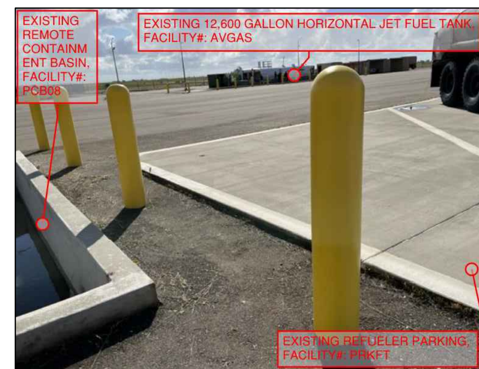
A14 EXISTING REFUELER PARKING PAD (LOOKING SOUTHEAST) SCALE: NO SCALE
