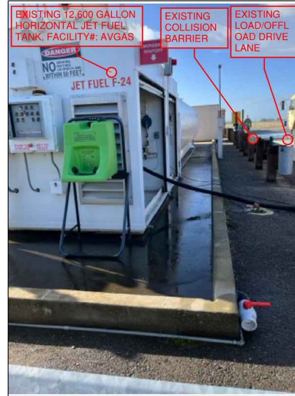
J11 EXISTING ASPHALT PAVEMENT BETWEEN TANK AND OFFLOAD/LOAD STAND (LOOKING SOUTH) SCALE: NO SCALE
