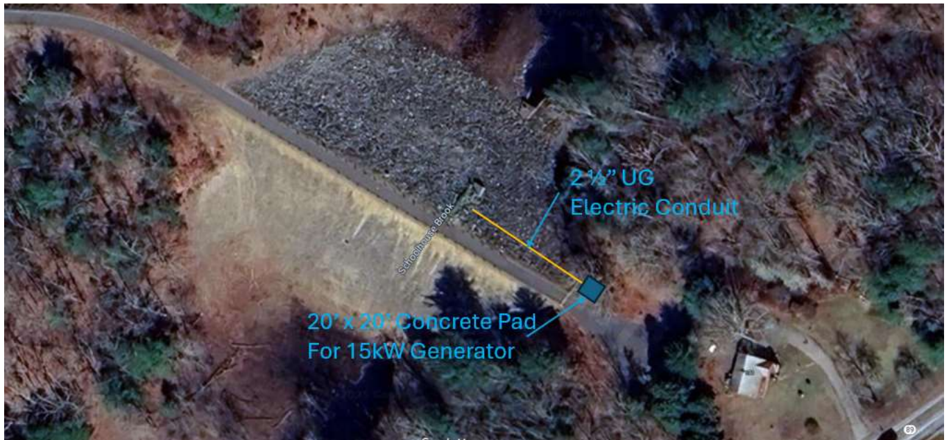
Image 1 : Aerial photo showing where concrete pad is to be placed and where existing underground conduit is.
