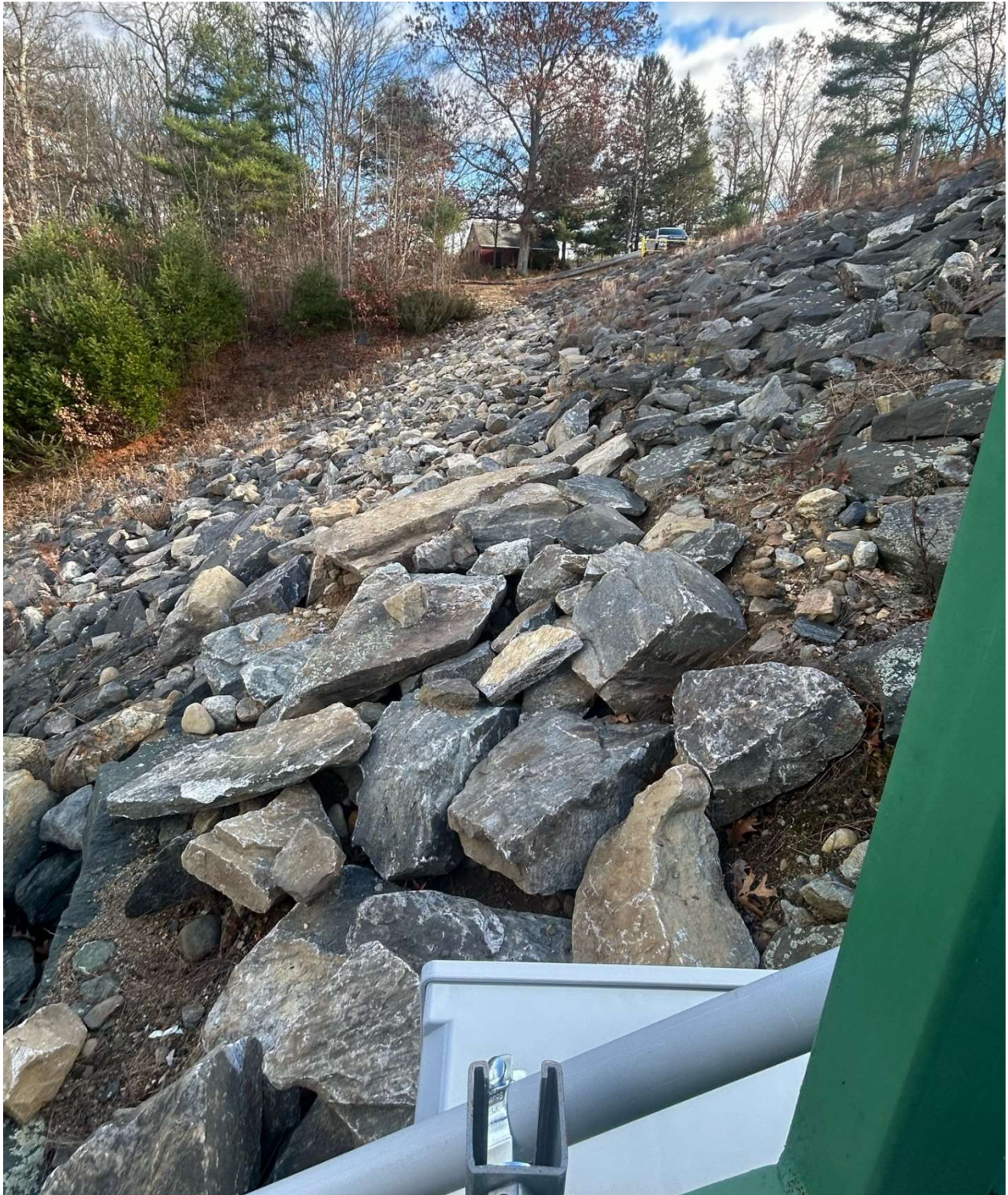
Image 6: Photo showing the pull box on the stairs and the run to the generator pull box.
