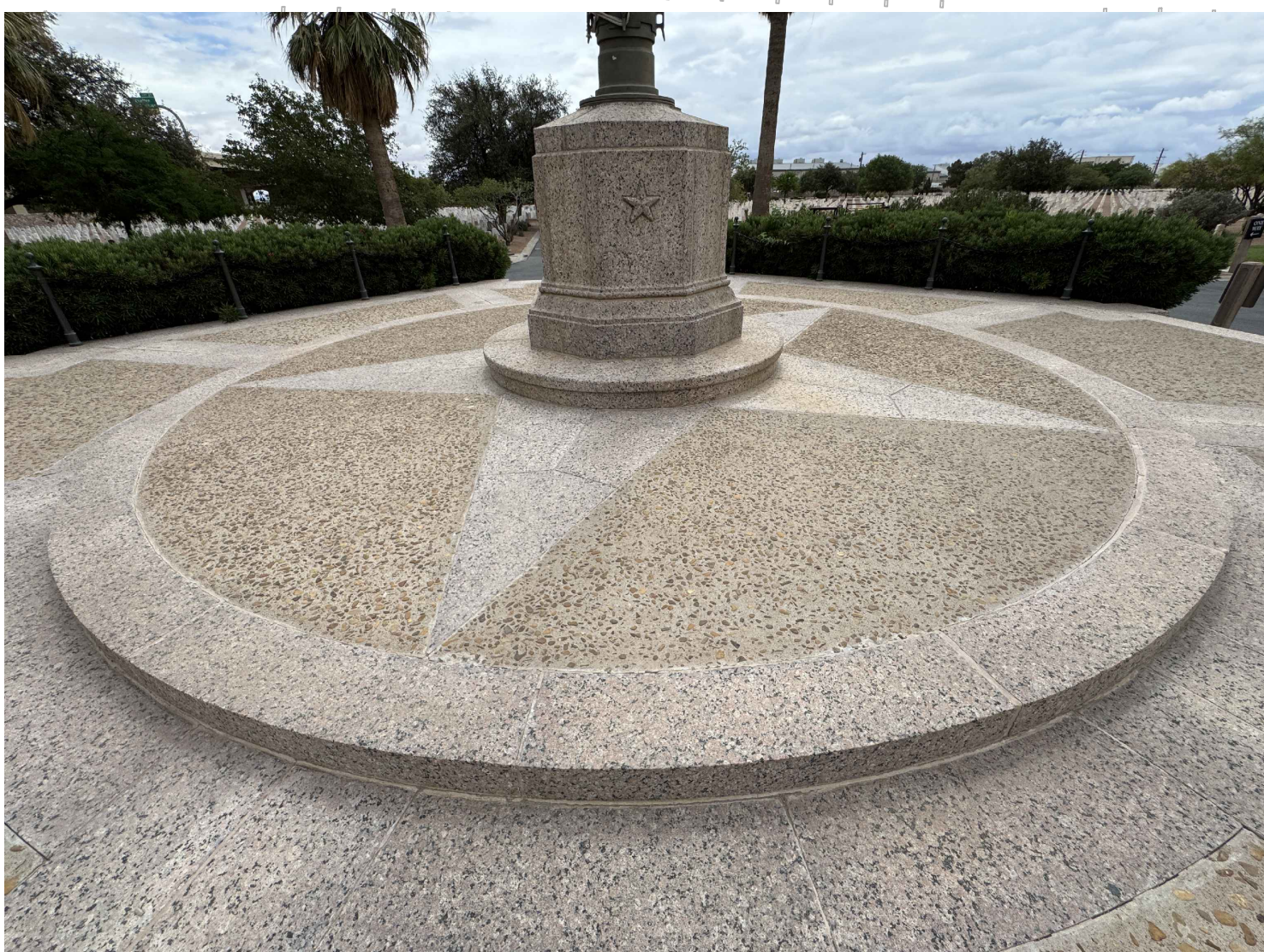
4 PHOTO DETAIL - FLAG POLE JOINTING
