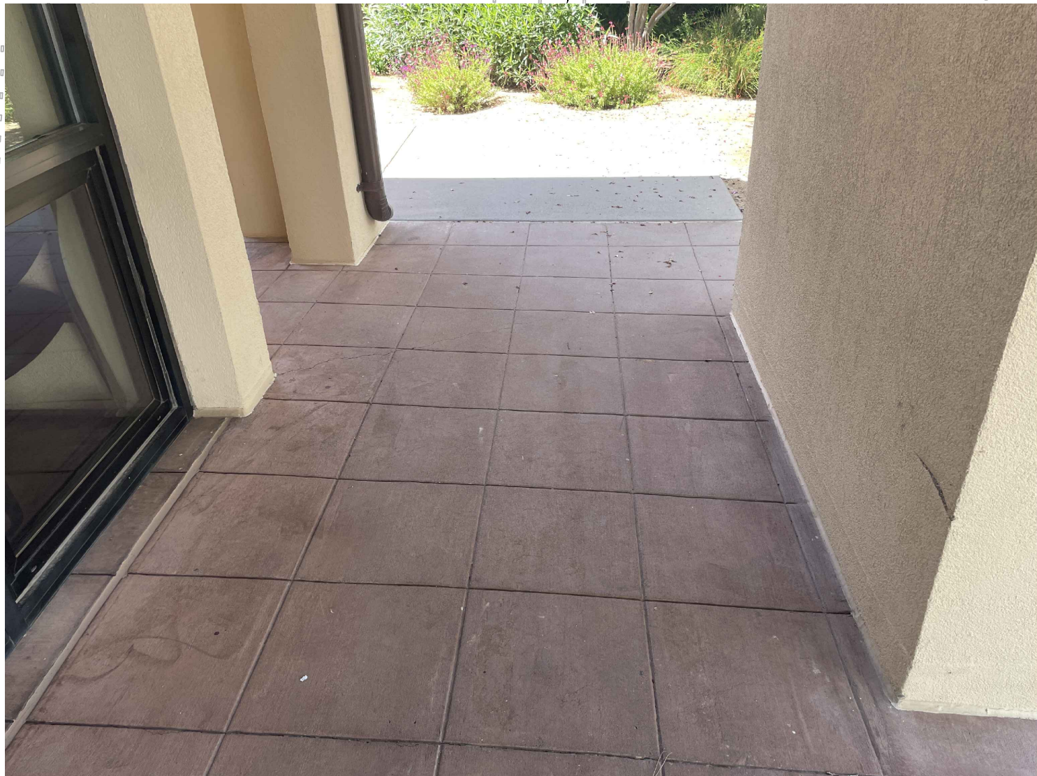
2 PHOTO DETAIL - STAMPED COLOR CONCRETE
