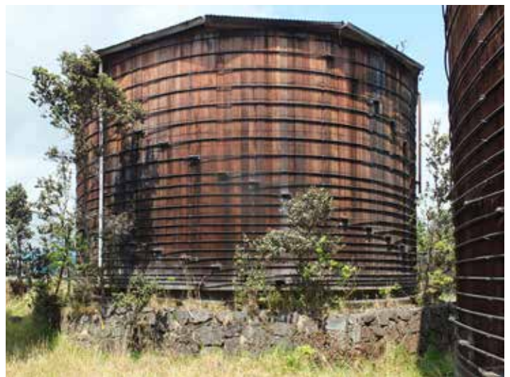
Figure 10: Tank 8 sits on an earthen platform retained by a rubble stone wall
