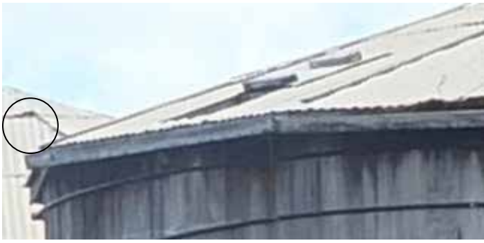
Figure 21: Tank 7 has an access hatch through the roof to provide entry to the tank interior. Logically every tank would need such a hatch. It may be that other hatches are not visible because they are closed (this hatch is open), and/or because they were not located in a position where the viewing angle allowed them to be seen from the ground. The corrugated aluminum roofing panels appear to be a light gauge and some may be working loose (circled).
