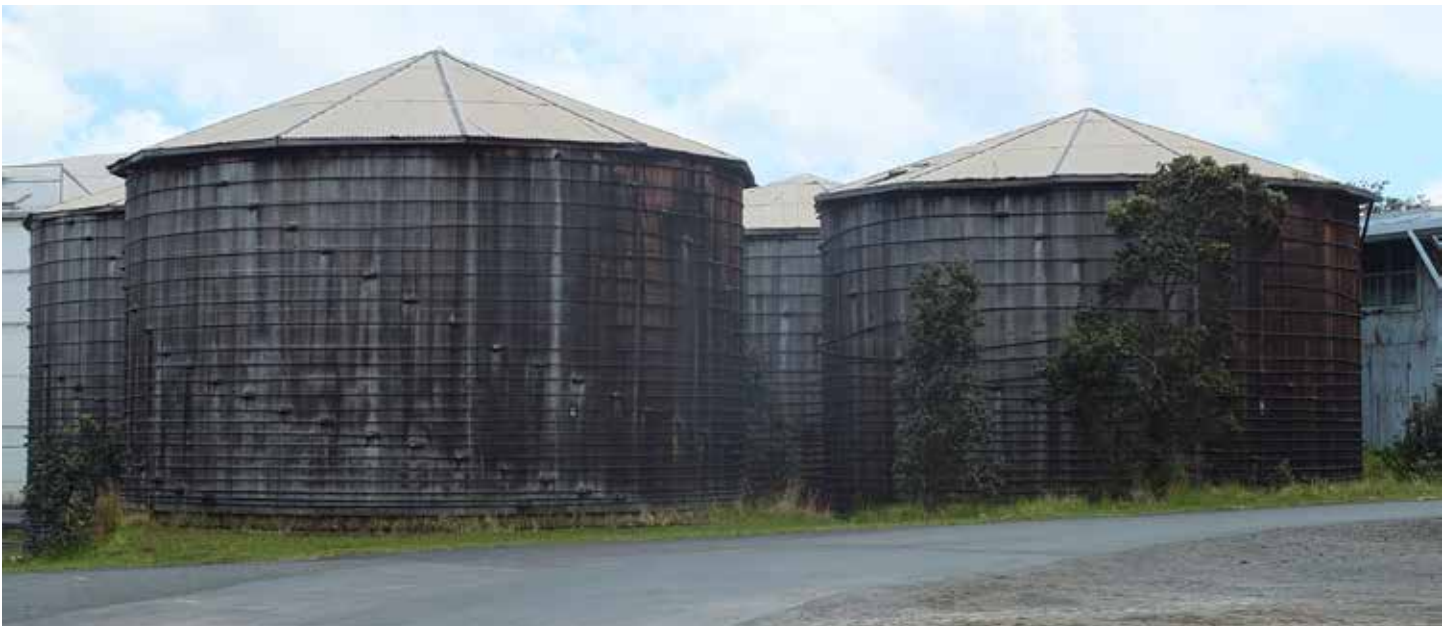
Figure 2: General view of the remaining redwood tanks. The tanks all hold 100,000 gallons except the tank on the front left which is smaller than the others, holding only 80,000 gallons.
