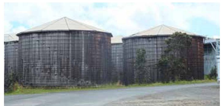
Figure 20: Each tank has a 12-sided pyramidal roof that is covered with white corrugated metal panels. The tanks originally had wood gutters, sections of which remain on some tanks.
