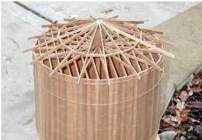
Figure 25: Although a scale model, this shows a tank with both a conical roof and framing that is flush with the top of the tank. Framing of this type, if it exists in the HAVO tanks, would help to prevent the inward collapse of the staves.
