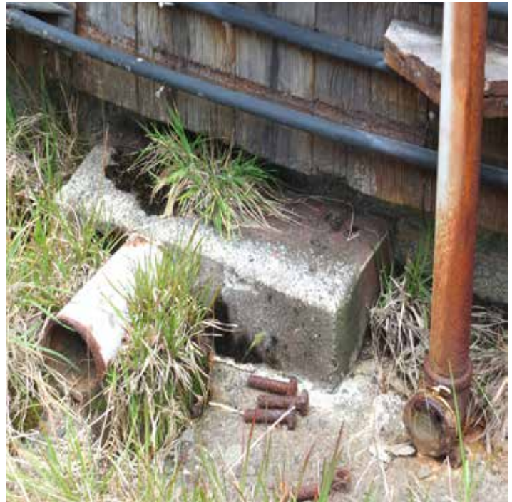
Figure 27: Existing internal drains or exterior pipes could be utilized in place of a traditional downspout to carry the water collected by the gutters down to the ground. How this is accomplished will need to be determined on-site, based on actual conditions.
