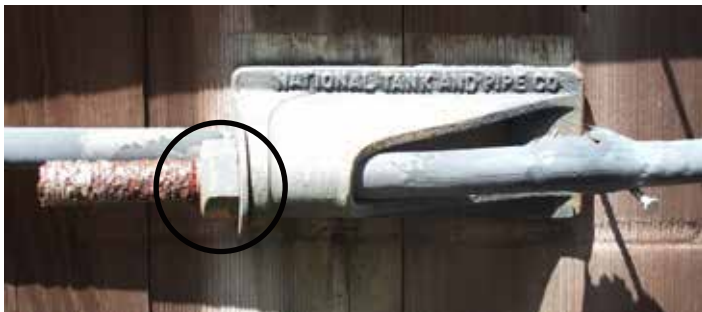
Figure 5: Close-up view of one of the lugs that connects the 5 sections of each steel band. The threaded connection with the nut (circled) allows the bands to be tensioned so that they compress the wood staves and resist the outward thrust of the water.
