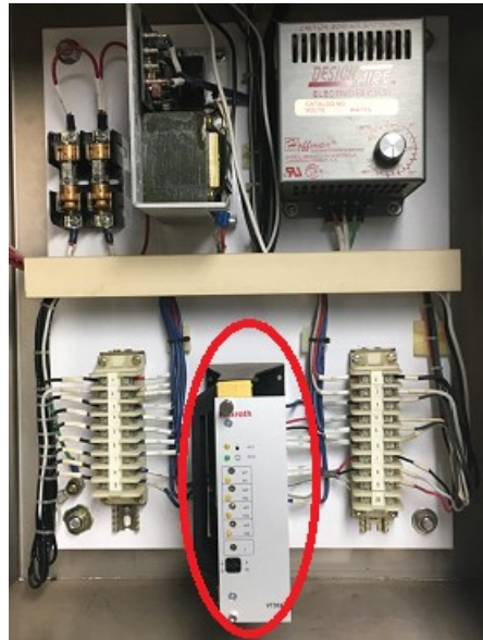
FIGURE 3. CARD AND HOLDER MOUNTING POSITION
