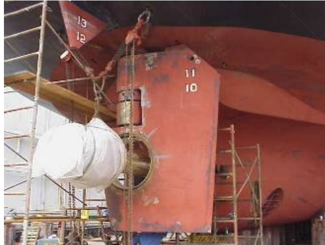
FIGURE 1. PHOTOGRAPH OF SHAFTING BEING REMOVED THROUGH RUDDER
