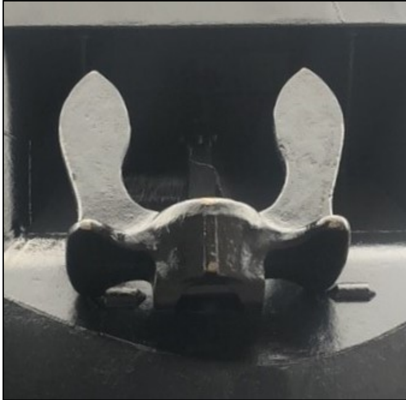
PHOTO 1: EXISTING TRIPPING BRACKETS (STBD SHOWN)
