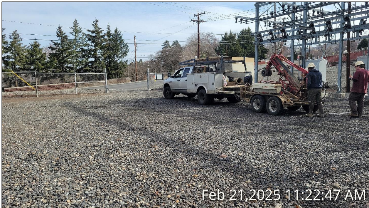
Photo 3: Drill rig setup at exploration location B-1, looking northwest.
