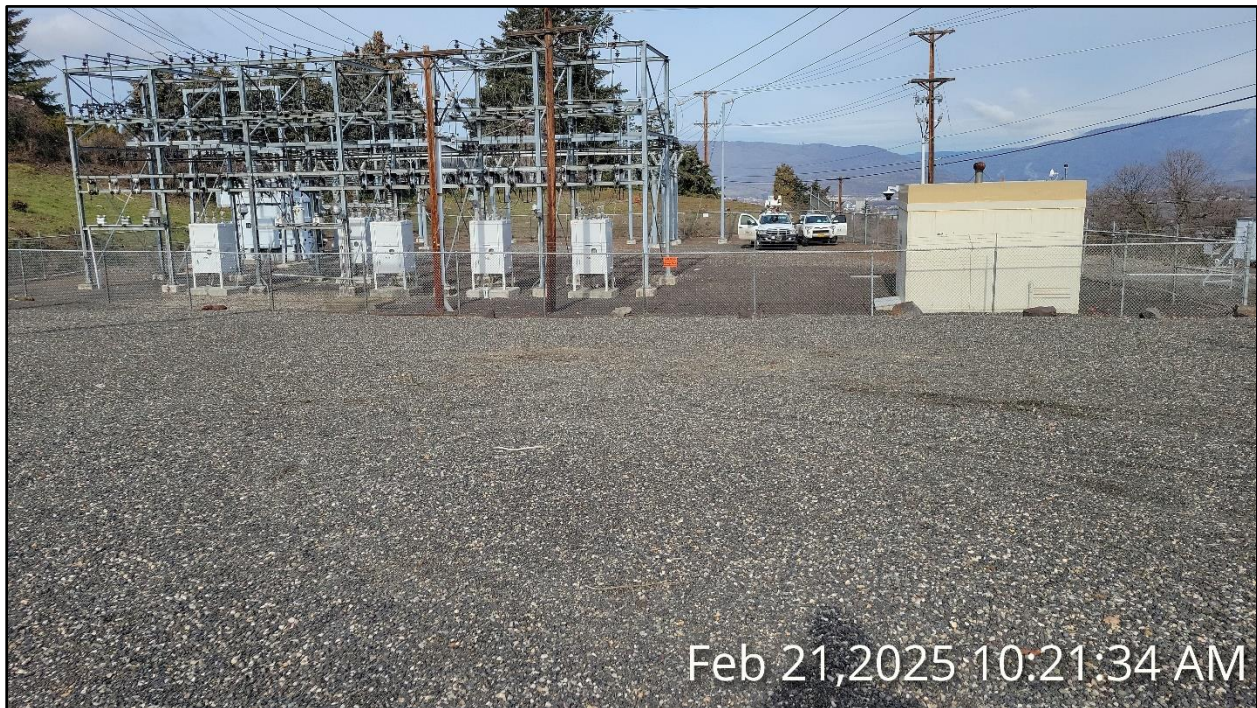
Photo 2: Site conditions at the time of our investigation, looking west from the eastern portion of the property.
