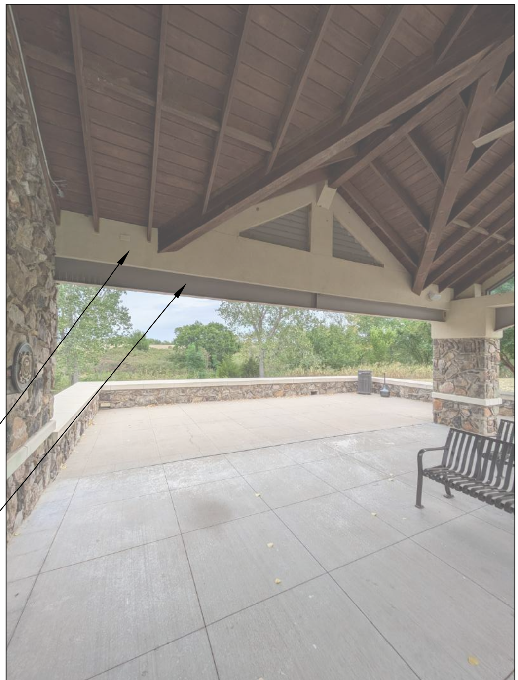
D7 IMAGE VIEW OF THE SHELTER ROOF SCALE: N.T.S
