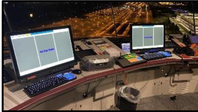
TFDM Controller Workstations with Touchscreen Displays
