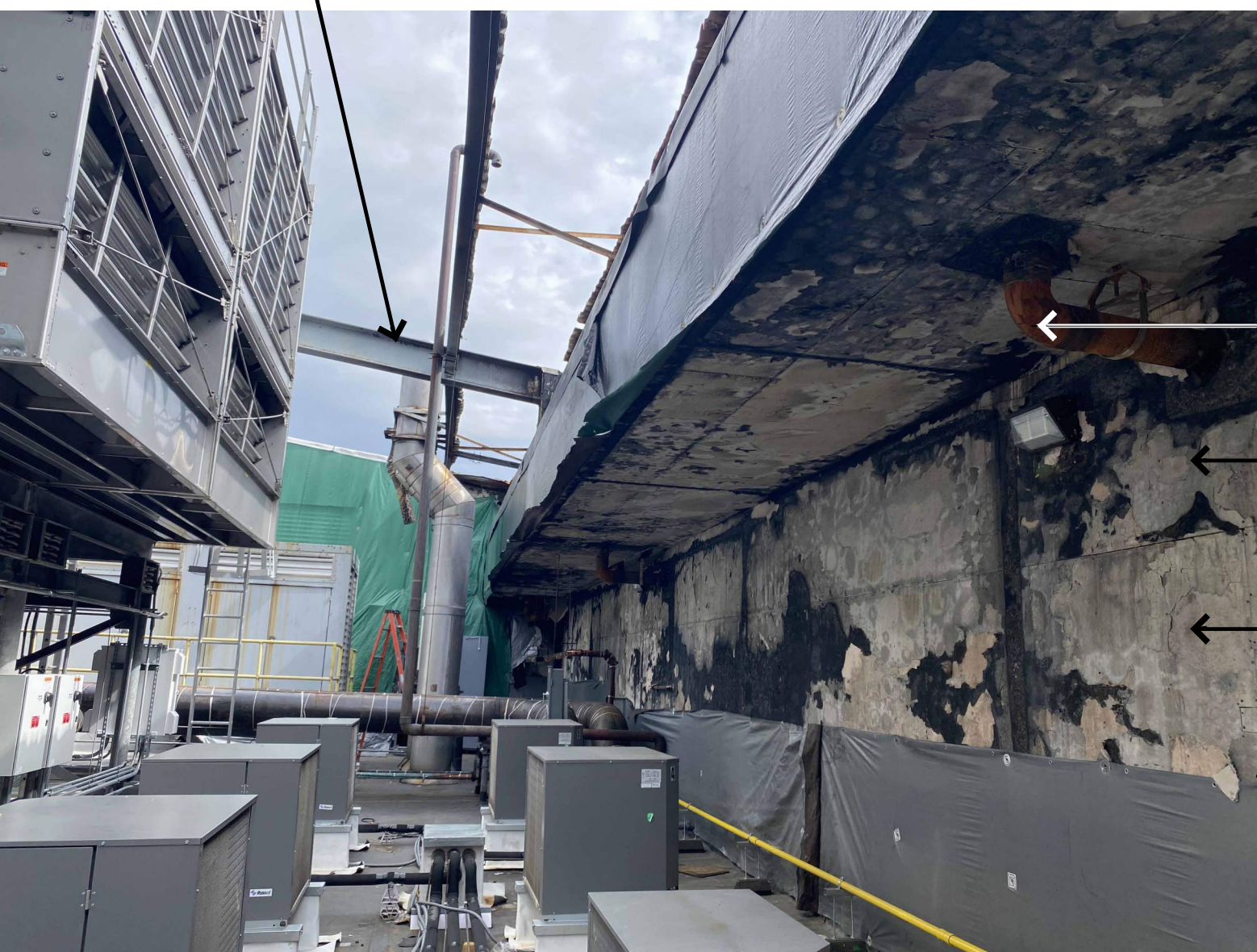
UNDERSIDE OF GUTTER
