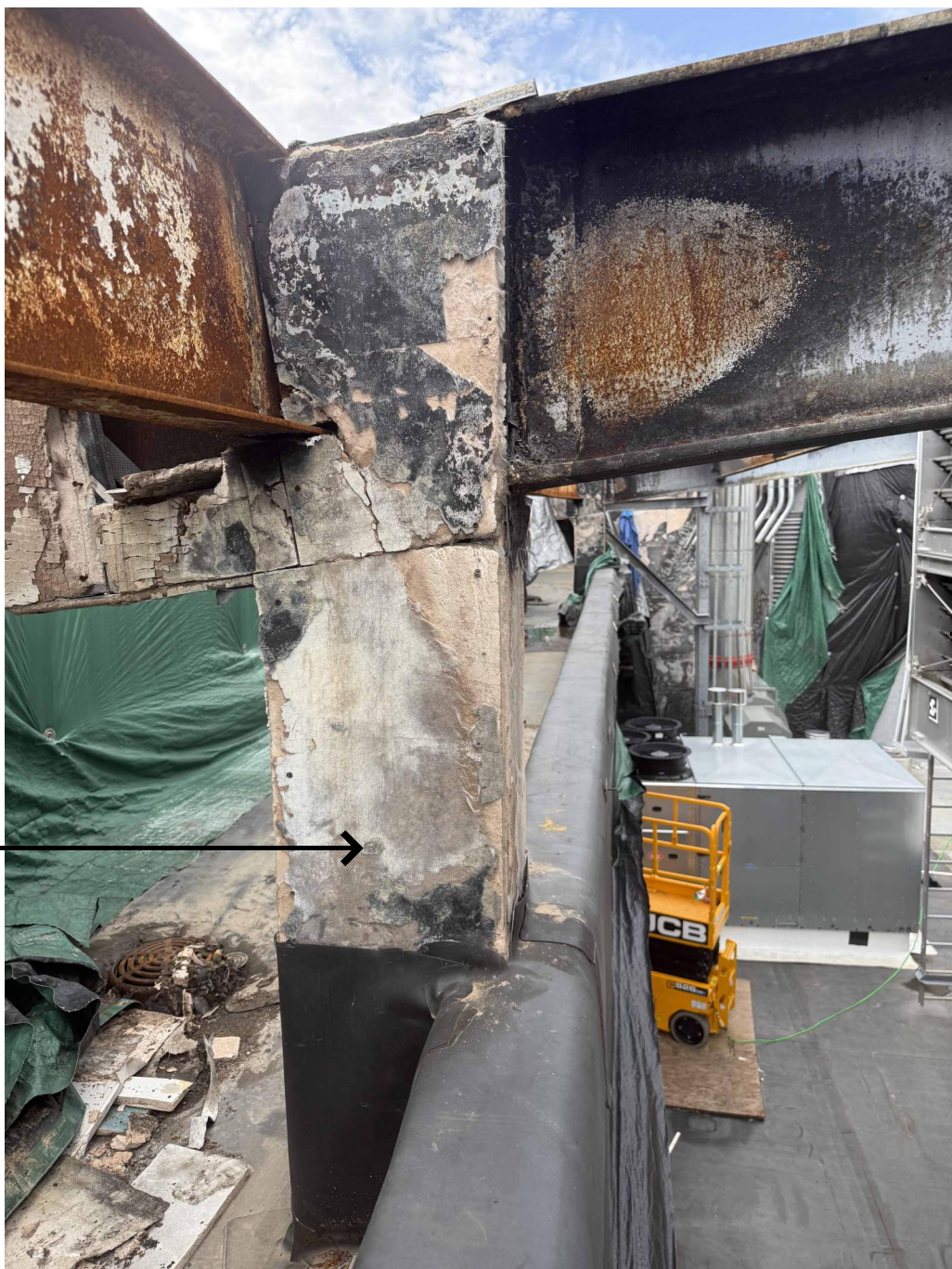
STUB COLUMN AT GUTTER TO FLYING BEAM
