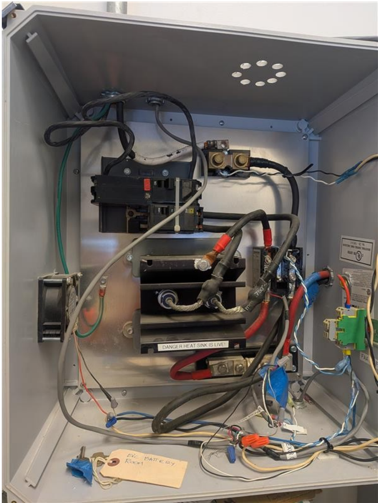
Photo 2 - Interior of the upper-left equipment enclosure, as identified in the A/E field notes. Specific equipment function and existing connections shall be field verified.
