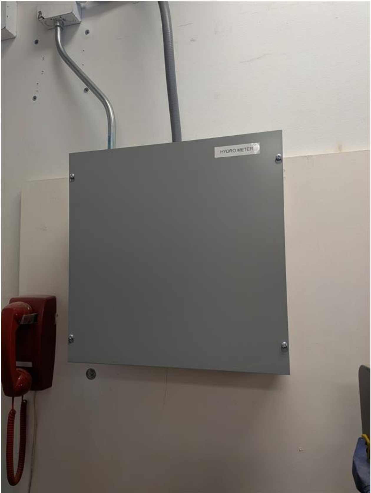
Photo 4 - Upper-right enclosure labeled "HYDRO METER." The interior of this enclosure was not photographed.
